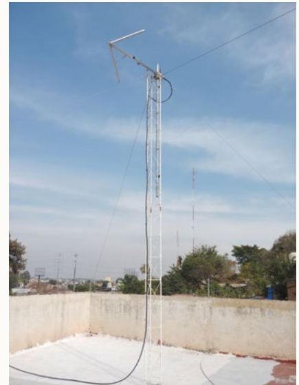
Radio antenna on the roof of the radio station.
