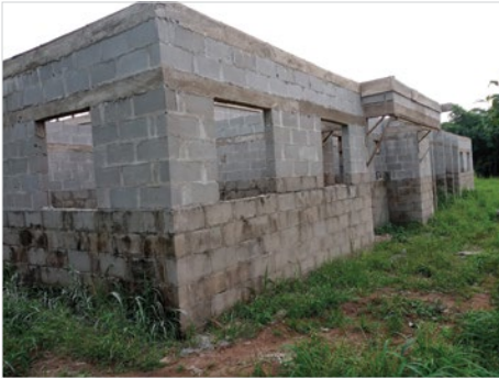
Ready for roof and windows.
