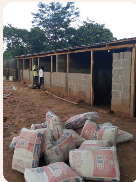
School classrooms being built at Apir
